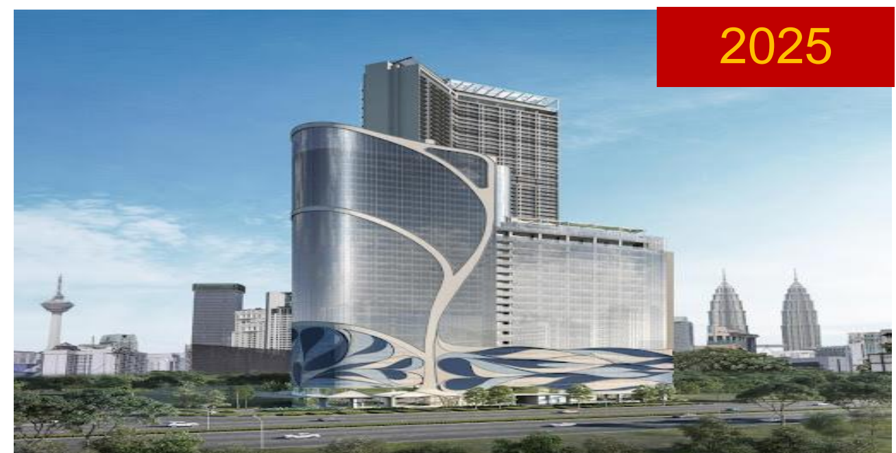
KL City | Adjacent TRX, Jalan Tun Razak Multibay 28 storey office tower
